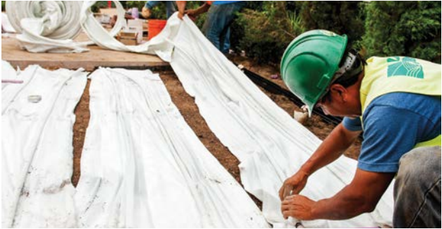
Eco-Mat instalado
